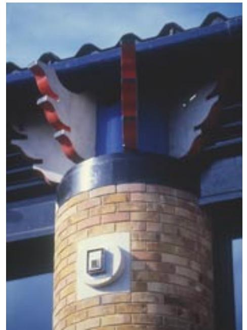
The Capitals of what we termed our 'Working Order', were polychrome from their beginnings in the Harp Heating Building in 1982-'85.
